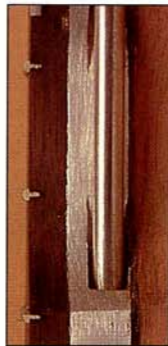
Alvarez steel truss-rod/magnesium U-channel in the neck.
